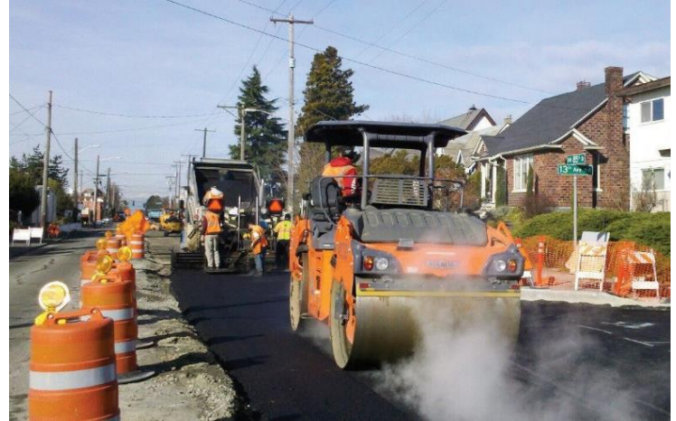
Example of crews paving the street
