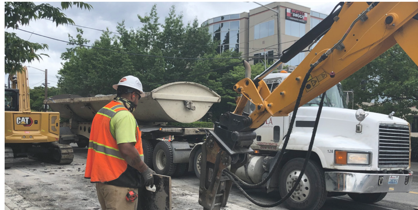
Construction worker prepares the roadway for resurfacing
