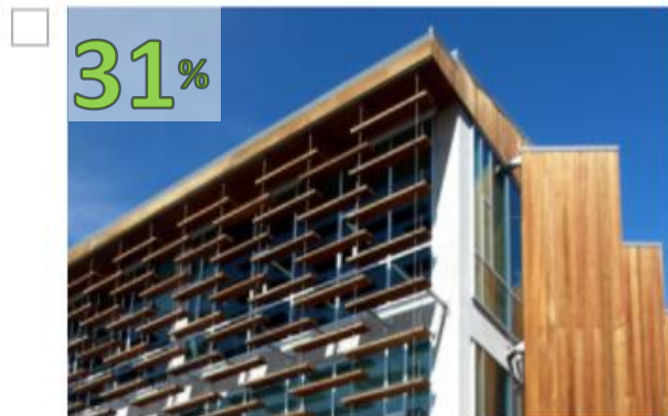
E. Details that add interest to this facade include energy-saving wooden louvers and shutters.
