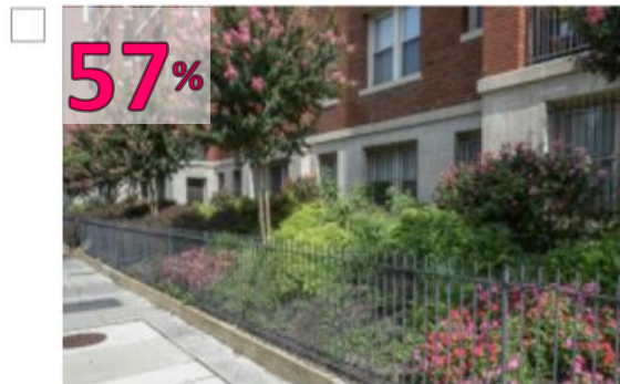
B. Multi-family residential buildings with a deep setback, fencing, and dense and colorful landscaping adds privacy for street level units.
