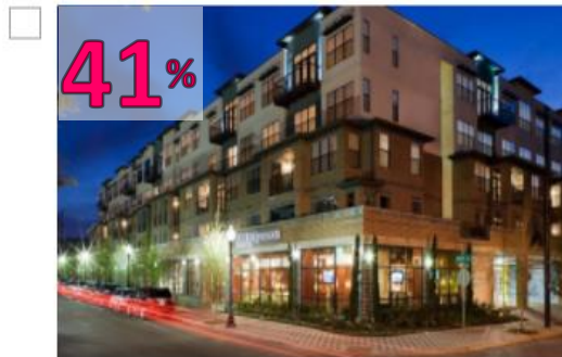
E. Complex building volume with distinct base, middle, and top. Balconies, bays, and strong horizontal cornices add detail to the building mass.
