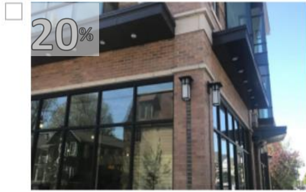
D. Facade details include contrast between dark glass, brick pattern, pedestrian lighting, and canopy with recessed lighting.
