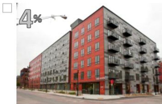
F. Consistent, simple materials with contrasting color to break down a block-long building facade.
