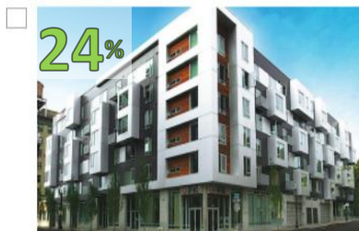
F. Simple building volume with highly articulated forms at the corner, and window bays applied in an asymmetrical pattern.
