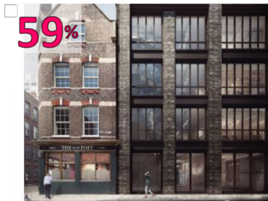
B. New building borrows proportions and materials of adjacent character building.
