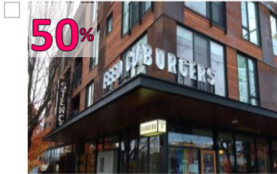
D. Combination of wood planks and rusted metal panels on upper floors. Glass, wood and other details add interest ground level.
