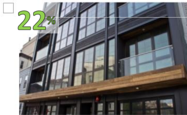
F. Details that add contrast to this facade include mix of contemporary materials--glass, metal, stained wood and a natural wood canopy.
