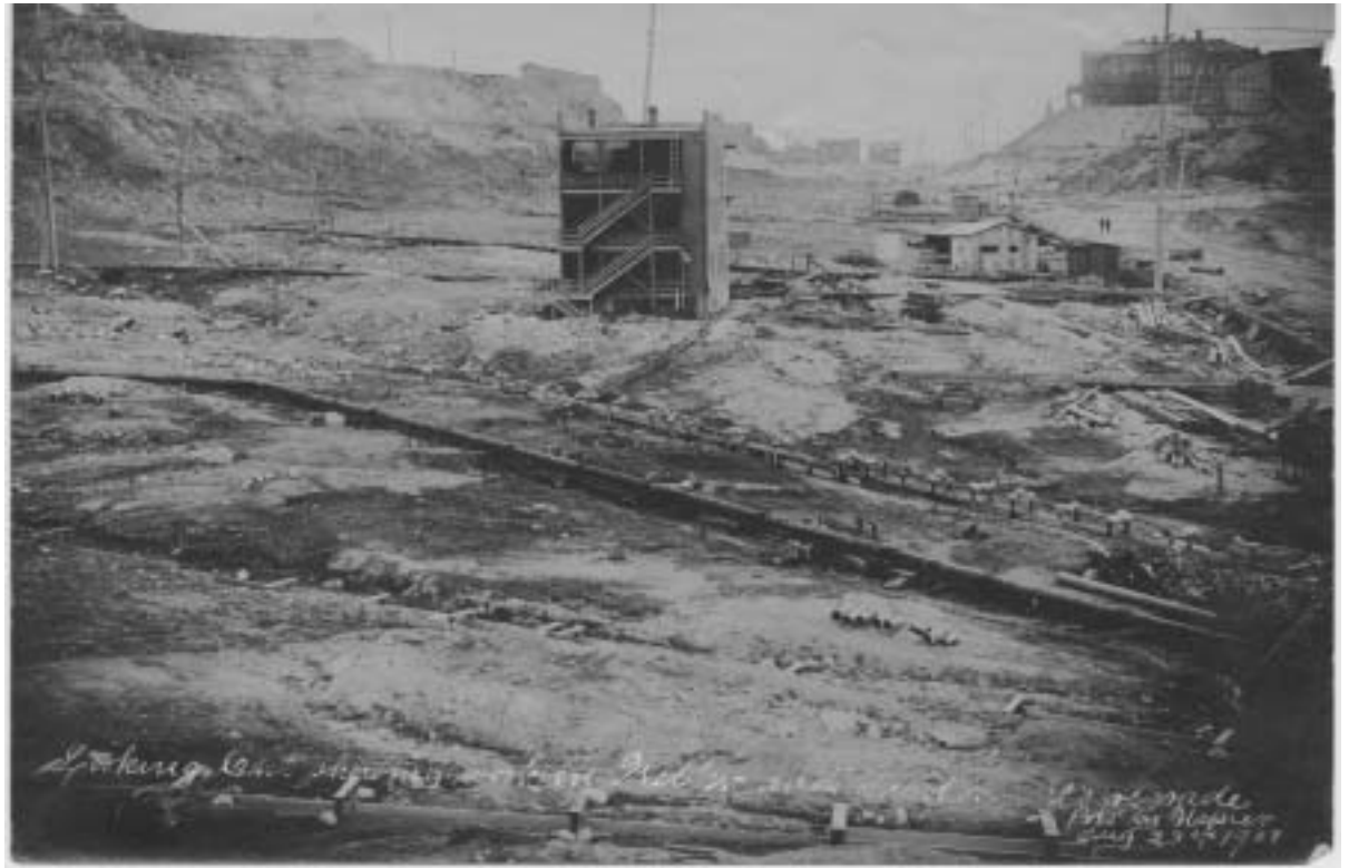
Dearborn Street under construction in 1909. Source: Rainier Valley Historical Society.
