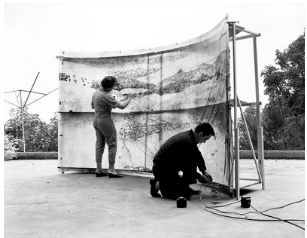
Installation of Electric Pavilion Mural, April 1962 Item 165730, Seattle Municipal Archives
