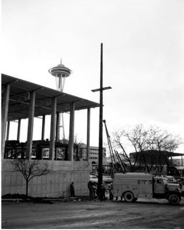
Removing last utility pole on Fair Grounds, October 1961 Item 165678, Seattle Municipal Archives
