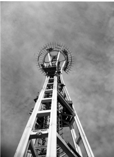
Space Needle construction, November 1961 Item 165649, Seattle Municipal Archives
